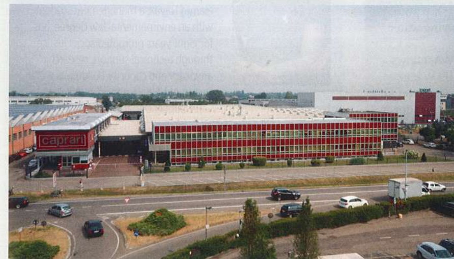
Caprari's headquarters in Modena, Italy
