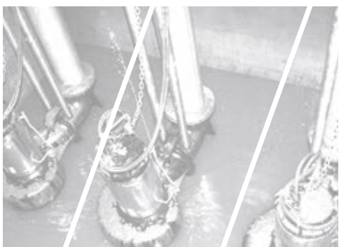
Wastewater Transport and Treatment
